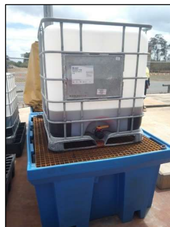
Photo 6: portable bund for a 1,000L IBC.
